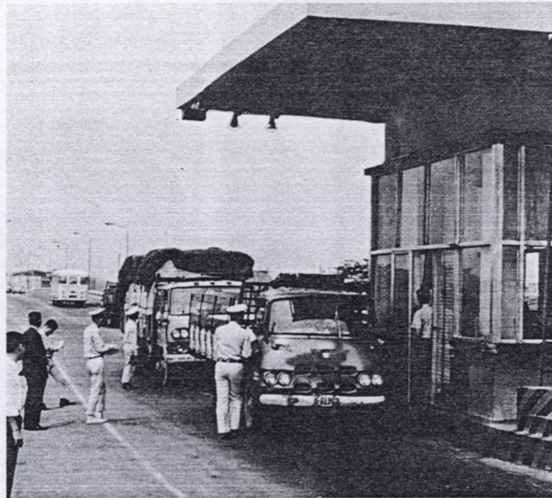
McArthur Thruway Toll Plaza
